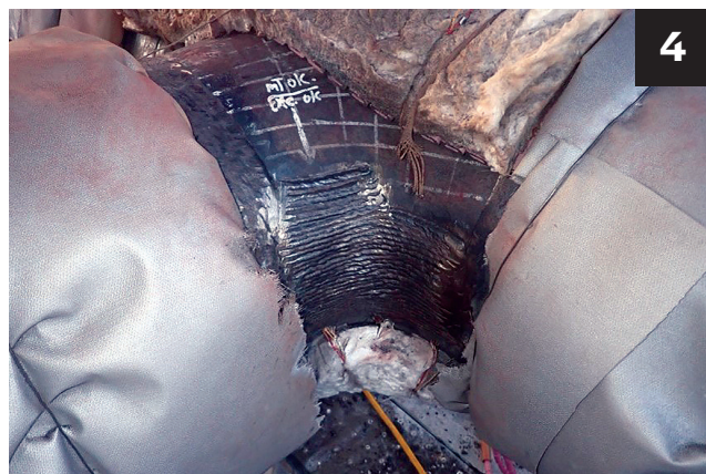
Fig. 4 — This crack was found using phased array ultrasonic testing (PAUT). Once plotted, a repair plan was developed and the welders excavated the crack to just before breaking the system open. Preheat was applied and the weld repair began until flush with the contour of the tee. (Photo credit: Combustion Engineering Solutions [CES-ATC].)
