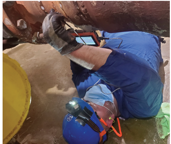
War2In graduate William Gollhofer performs UT to detect fluid-actuated corrosion on 20-in. main-steam piping at the Byron Nuclear Power Facility in Byron, Ill.
