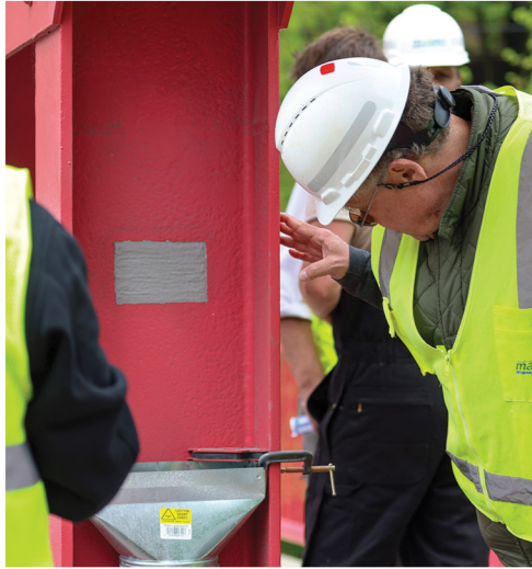
Fig. 2 — The first field demonstration of cold spray additive repair on a steel bridge in Great Barrington, Mass. The project included repair of a corroded steel girder; inspection of the completed deposition; and collaboration among researchers, MassDOT engineers, and industry partners. (Credit: UMass Amherst.)
