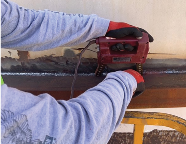
Magnetic particle testing on an above-ground storage tank in Long Beach, Calif.
