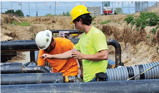
Devon Morr (right) looks at pipes on a job site.
