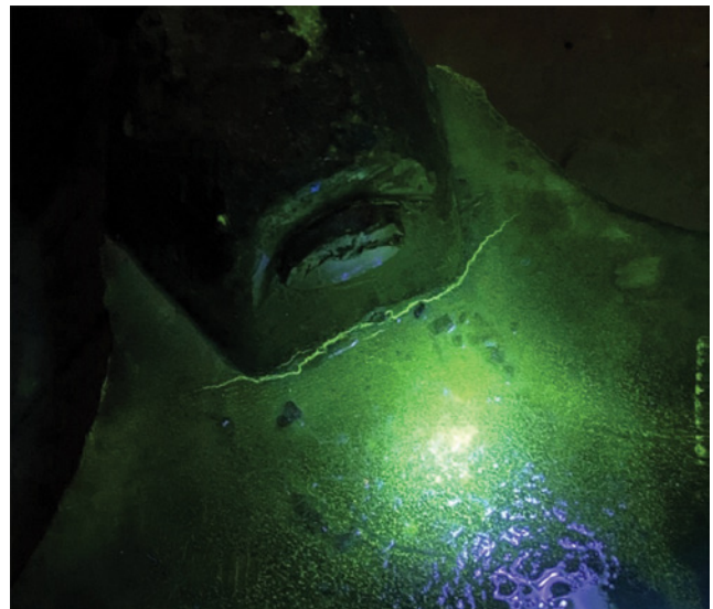
Fig. 2 — In-service crack on a critical member of a carousel-style ride using wet fluorescent MT.
