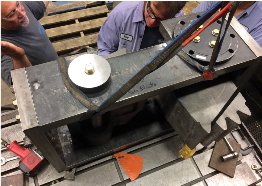
Fig. 3 — This photo shows the size of the part that has to be repaired by welding two pieces together. Notice the workers placing the two halves into the fixture and ensuring they are properly aligned.
