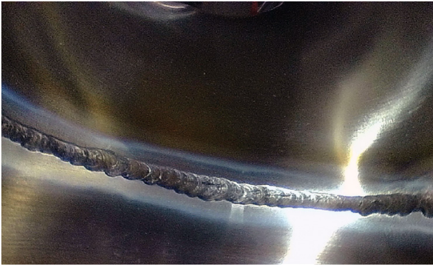
Fig. 1 – A borescope image showing excessive lighting, causing blooming.
