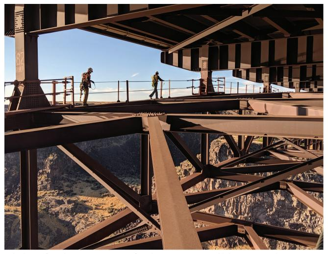
Wheeless performed corrosion assessment of weathering steel, coring, and bolt extraction at the Perrine Bridge in Idaho.
