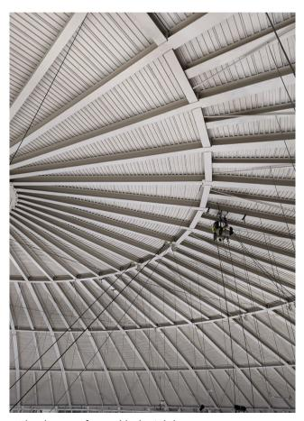
Wheeless performed industrial rope access techniques to install structural supports to be used for new sound equipment at the Purdue University Mackey Arena in Indiana.
