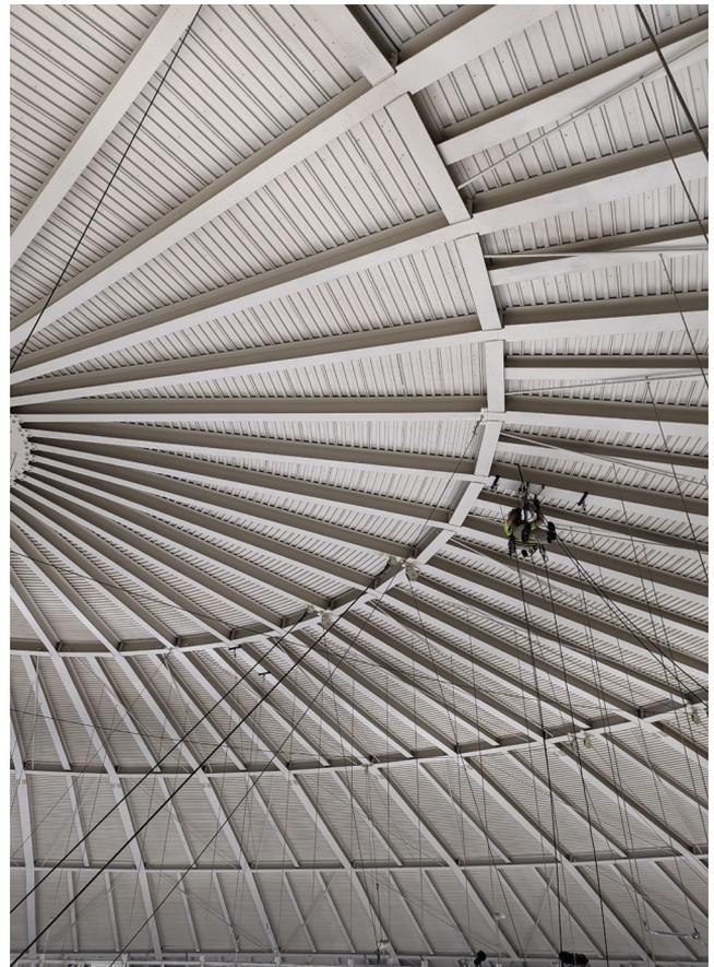
*Wheelless performed industrial rope access techniques to install structural supports to be used for new sound equipment at the Purdue University Mackey Arena in Indiana.*
