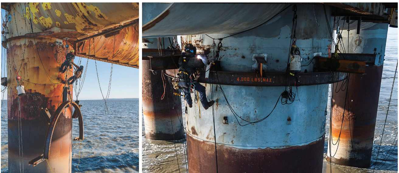
Welding and inspection using rope access in the offshore environment. (Photo courtesy of Rigging International Group.)
