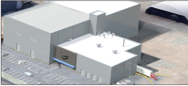
The Boeing Phantom Works Advanced Coatings Center in St. Louis will house postassembly phases of future military aircraft production (Boeing artist's concept).
